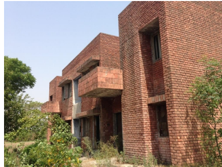
Staff Residence: External
