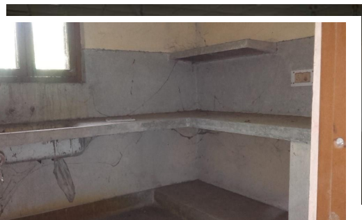
Staff Quarters: Internal
