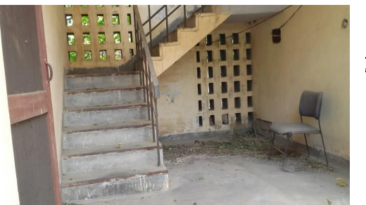
Staff Quarters: Internal
