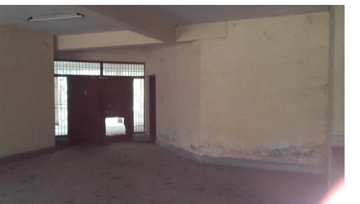
Staff Quarters: Internal
