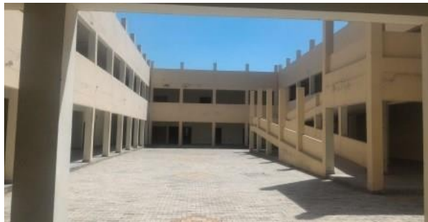
Main Building: Internal Courtyard
