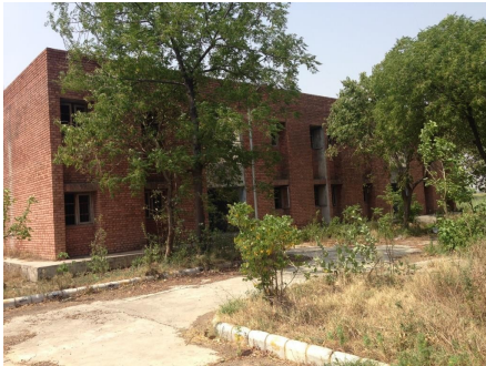
Staff Residence: External
