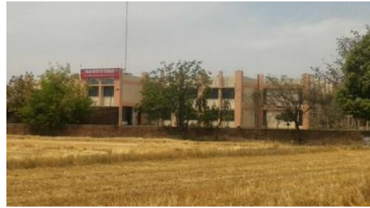
Existing Condition of the Site
