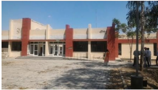
Building 2: External View
