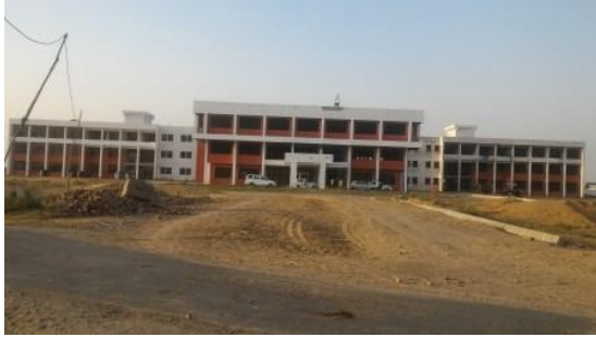
Building 1: Administrative Building
