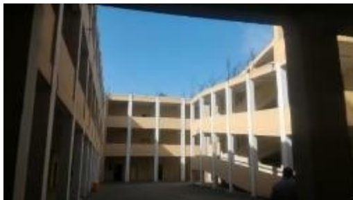
Main Building: Internal Courtyard
