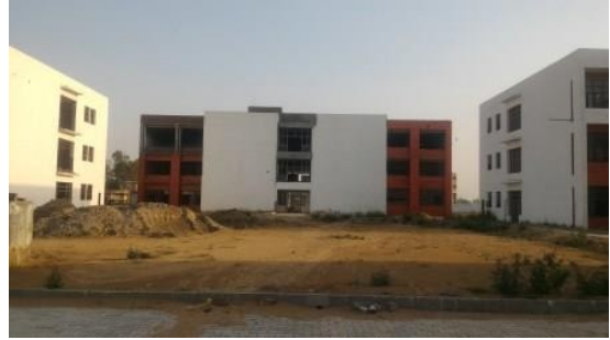
Building 1: Another View
