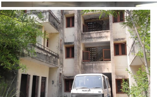
Staff Quarters: External
