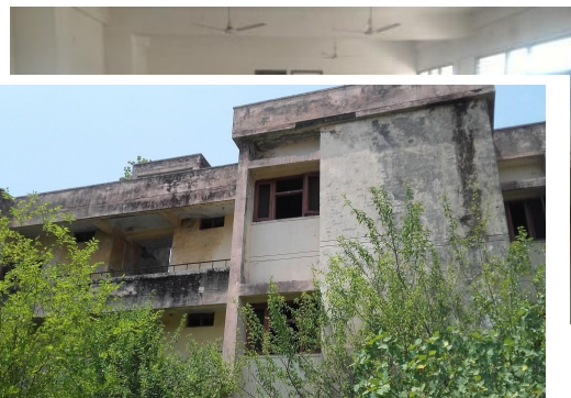
Staff Quarters: External
