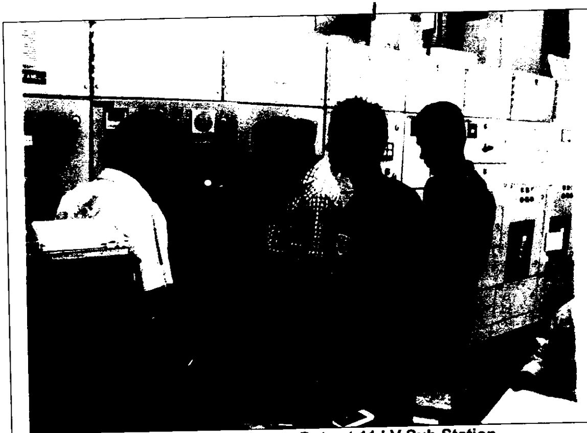
Measurement of Energy Data at 11 kV Sub Station
