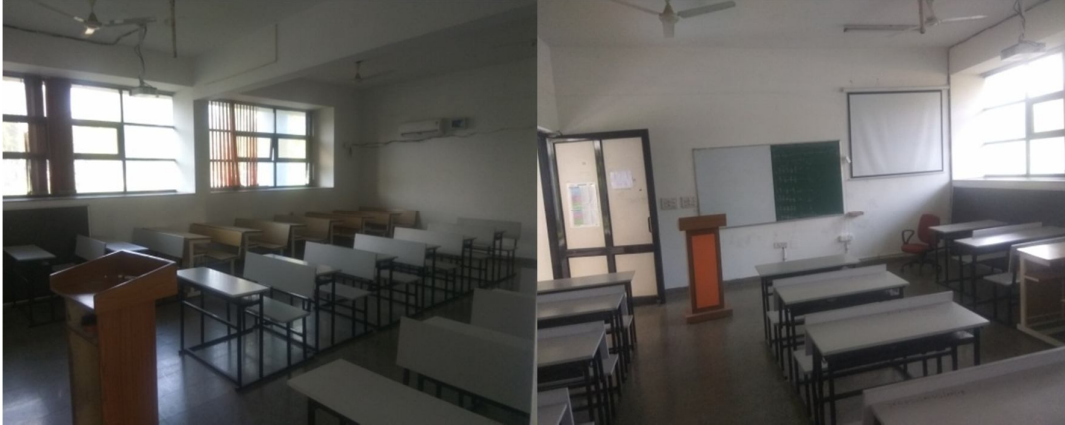
Day light and ventilation Condition
